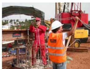
Installation of one of the removable extensometers
